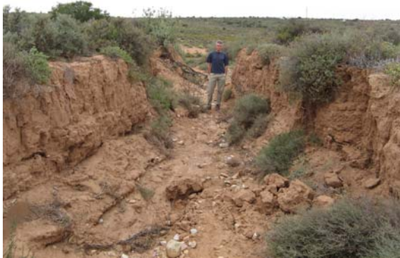
Before: Typical eroded donga system.
