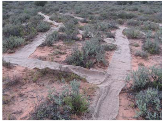
2. Jute geotextile ( Soilsaver ) is cut and laid along the paths.
