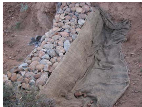
4. The upstream side of the gabion is then lined with geotextile to trap silt and fine plant material.
