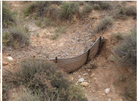
Fences with mulch check water flow and stabilize small dongas.
