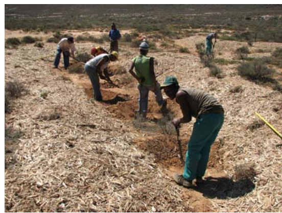
4. Reshaping and mulching of small dongas in between the sheet eroded areas.
