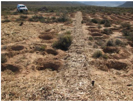
3. Erosion fences are added where the water flow must be checked.
