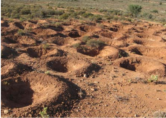
1. Hollows ( \pm 500 \times 500 \text{m} \times 200 \text{mm} deep) made across the bare area.
