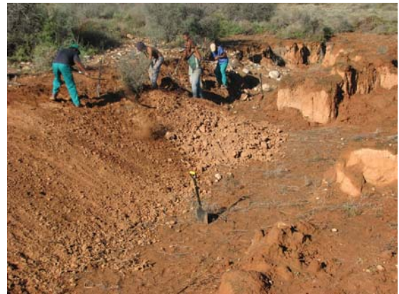
2. The gully sides are sloped by hand (or machine).
