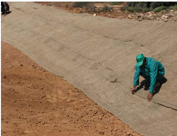
3. Jute geotextile ( Soilsaver ) is spread over and pinned onto the surface.
