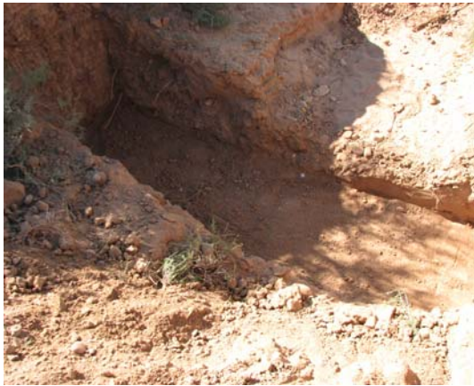
1. First a trench is dug into the donga floor and sides.
