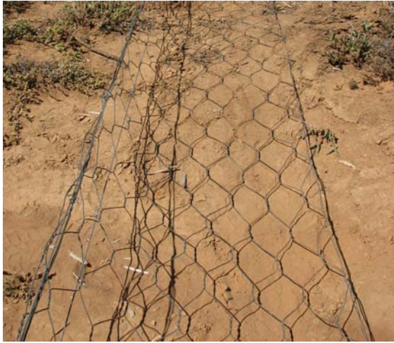
1. A sturdy low fence of iron standards and wire netting is made across the site.
