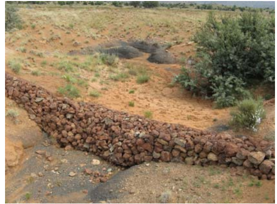
After: A functional stone gabion.
