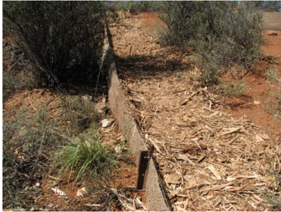
3. Geotextile should always be used together with wire netting.
