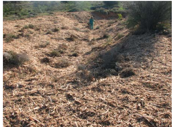
4. The entire shaped and stabilized area is then covered with mulch and seeded.
