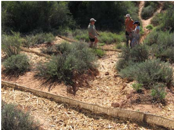
Fences can be used on slopes to treat small rills.
